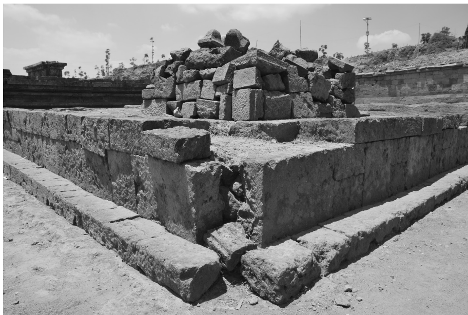
Fig. 7 – Candi Liangan, first courtyard. Batur 2a . Detail of the wall: stone blocks placed in shiner, infill of river stones and dirt. (Photography: V. Degroot)
