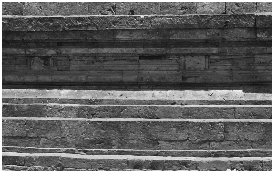
Fig. 6 – Candi Liangan, first courtyard. Candi nomor 1 . Detail of the wall: stone blocks placed in stretcher. (Photography: V. Degroot)
