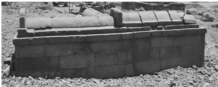
Fig. 10 – Candi Liangan, border of the second and third courtyard. Pagar lempeng batu , seen from the outside. Note the oblique junction between the first (to the left) and second (to the right) segments. (Photography: V. Degroot)
