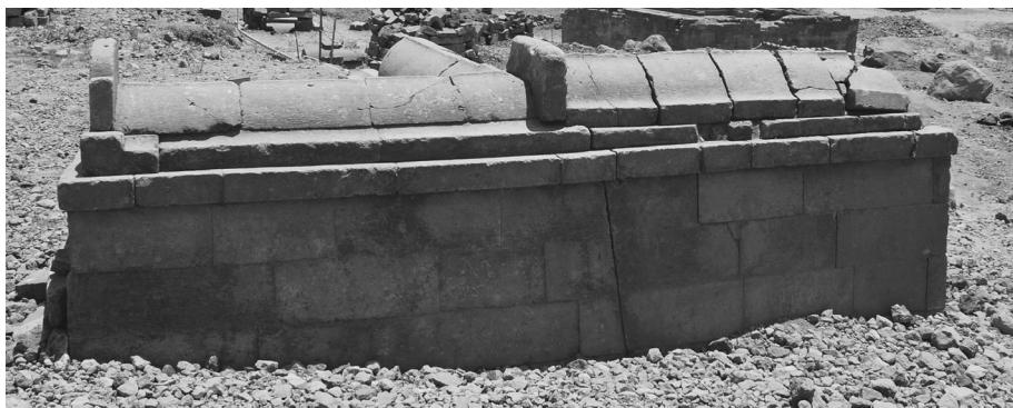
**Fig. 10** – Candi Liangan, border of the second and third courtyard. *Pagar lempeng batu*, seen from the outside. Note the oblique junction between the first (to the left) and second (to the right) segments.
