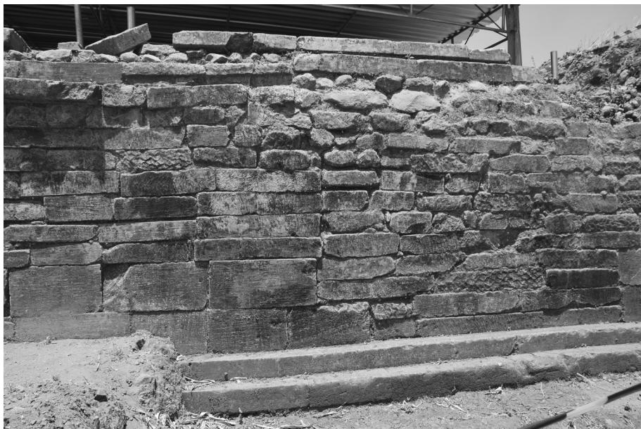
**Fig. 11** – Candi Liangan, retaining wall to the south of the first courtyard. At the bottom left, blocks placed in shiner. Elsewhere, stones placed in stretcher. Note the river stone (top right) and the blocks in reuse (top left), as well as the difference in surface finish. (Photography: V. Degroot)
